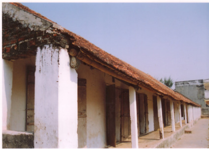
Old School Building
